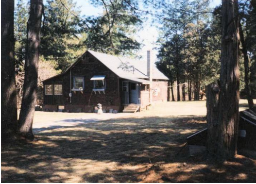
Cottage, 1995, from DCR CCC Archives
