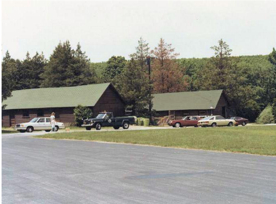
CCC Camp Buildings at Upton State Forest built in 1935
